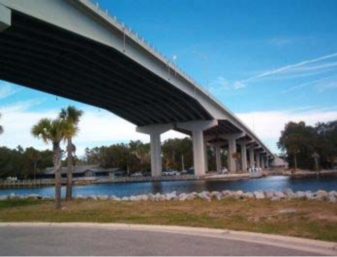
Bridge of Lions Restoration Miraculous Matanzas Inlet Palm Valley Bridge
